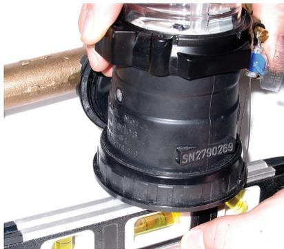
To tighten the locking nut, tighten counter clockwise.
